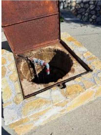
Figure 2.12: The installation well of the Komilio Station (System Number 5).
