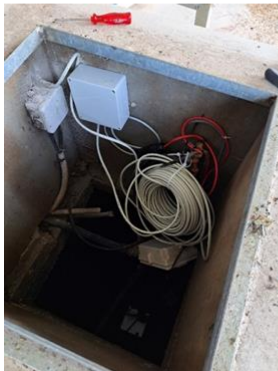
Figure 2.9: Transmitter unit of Brunello Station, as it was mounted onto the walls of the well.
