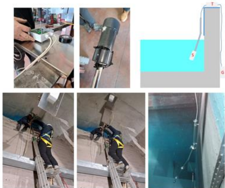
Figure 3.24: Sensor prototype installation characteristics of site 3 (SW Gran Sasso groundwater intake tunnels).
