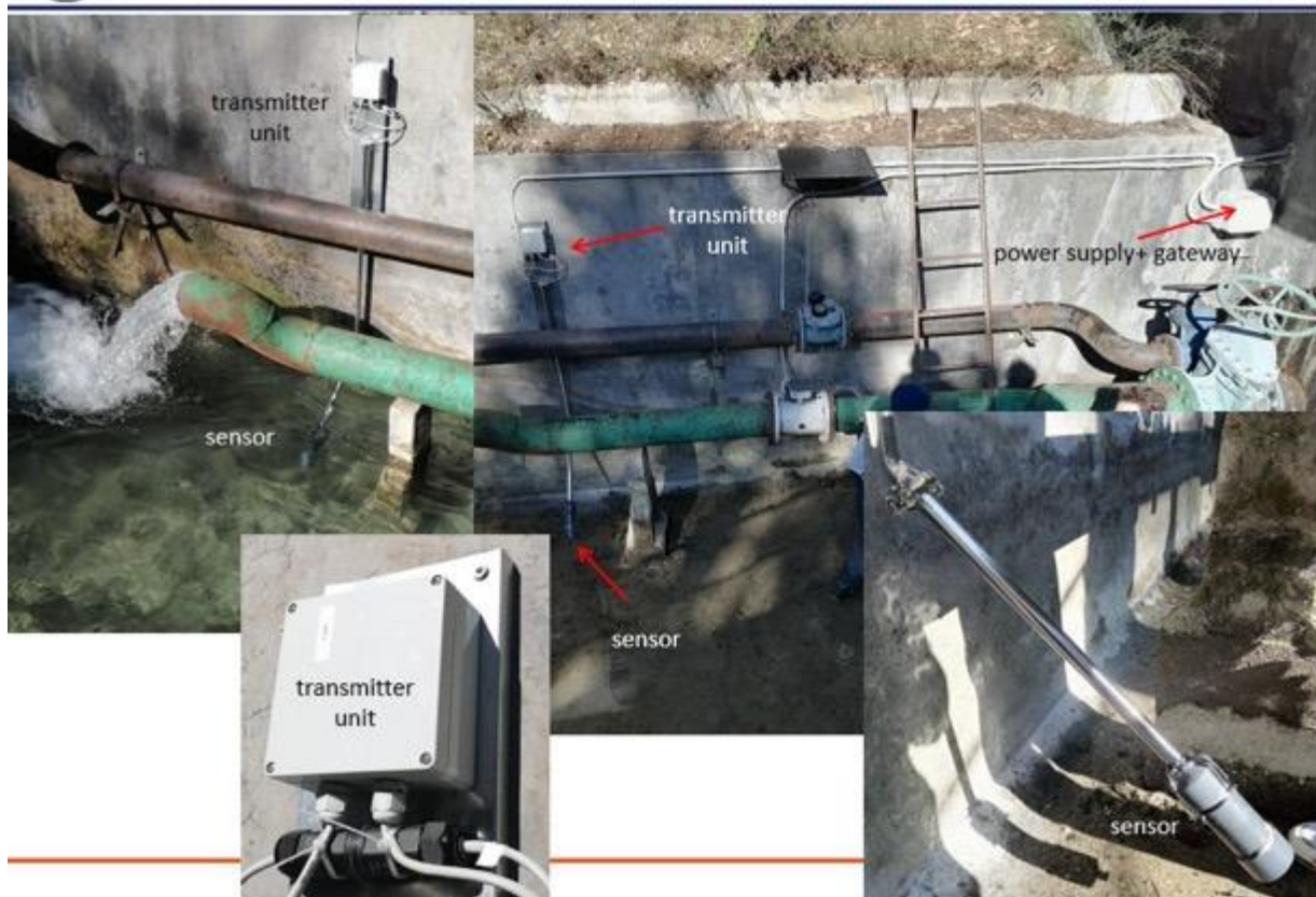
Figure 3.19: Giardino Spring (site 8). Sensor prototype installation scheme.
