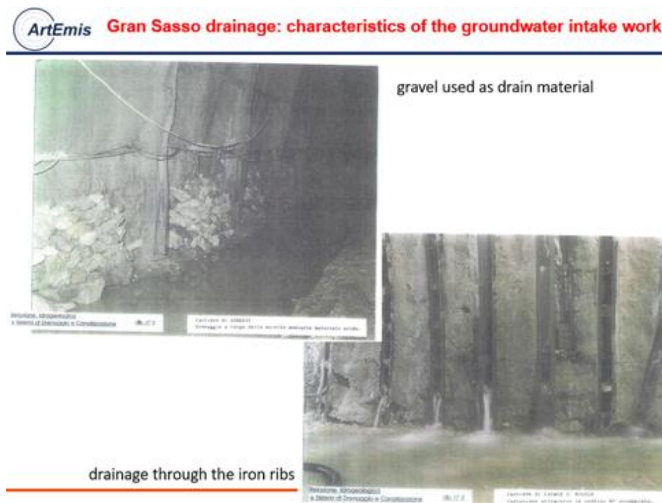
Figure 3.4: Withdrawal works in the tunnels for draining groundwater (Lunardi and Catalano, 1979).
